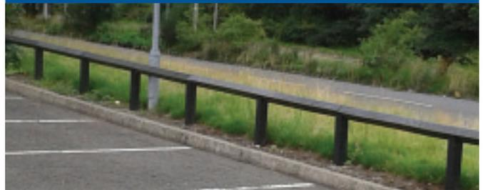
**Plastic Wood Rail:** A low level demarcation barrier constructed from recycled plastic, colour dyed to offer a highly durable 'timber like' fence .
